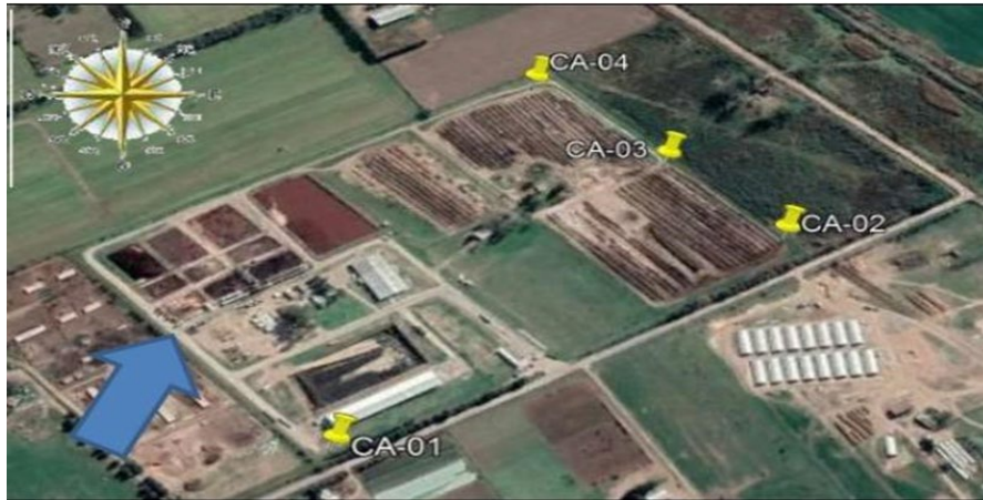
Figure 9. Monitoring positions for air quality at WORMS S.A. Source: Google Earth,
